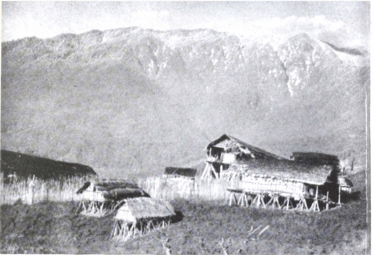
23. Dafa houses in Mengo village; in the background a 10,000-ft. ridge lightly sugared with new snow.
