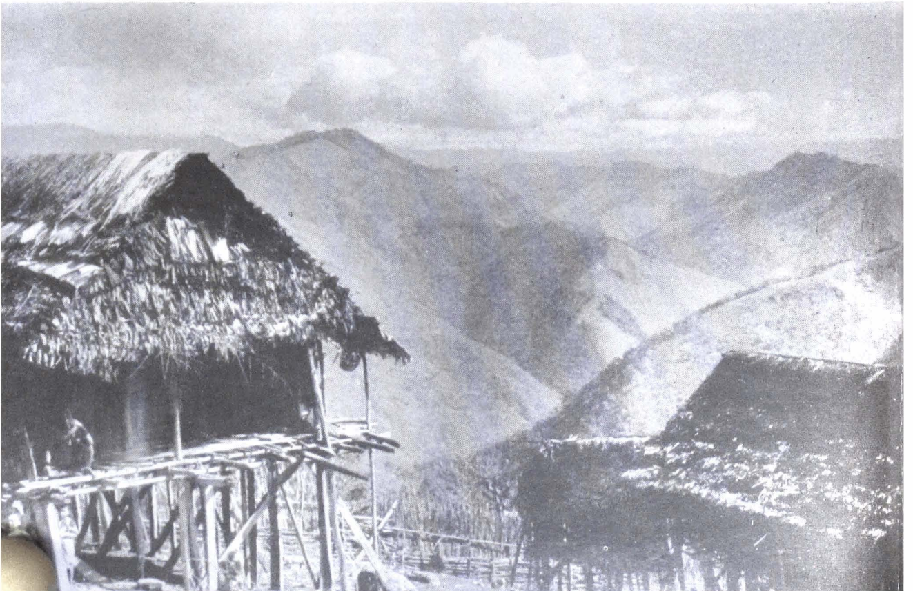
20. View over the Lower Kamla valley from Chemir village.
